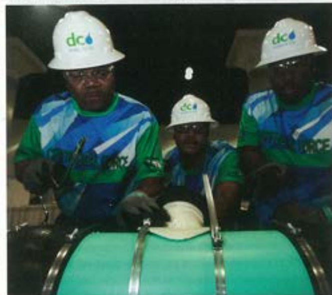
Moses Riley, Melvin Keys, and Aaron Montgomery, Centrifugal Force team members from the Chesapeake Water Environment Association, work to attach the service saddle on the replacement pipe. This year, in addition to the pipe repair, teams had to identify six pipe defects in a quiz. Kieffer Photography
