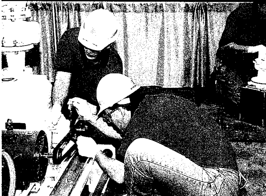
In the Maintenance Event, teams like Ohio's Main Drain, pictured here, replaced the belt of a centrifugal pump.
