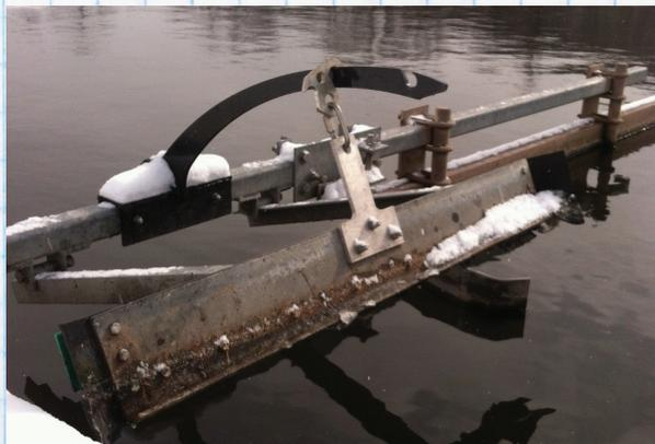
LIFTING THE SKIMMER ARM UP USING THIS HOOK PREVENTS IT FROM FREEZING TO THE TROUGH. THIS INGENIOUS FIX MAKES THE MOST OF EASILY AVAILABLE AND SAFE TOOLS AND IS QUICK, SAFE, AND SIMPLE TO USE. James Spielvogel
